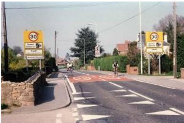
Figure 4: Gateway with speed limit change, dragons teeth marking, yellow backing boards for speed limit sign and speed roundels enhanced by coloured surfacing
